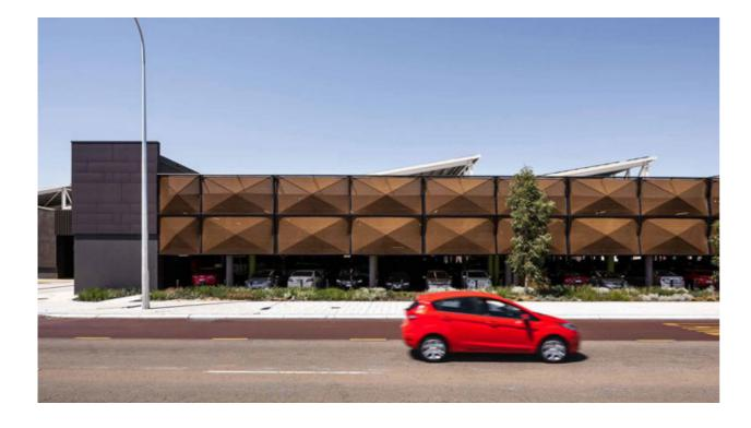
← LEFT: The threedimensional design is made up of a series of projecting pyramids which are stretched across a steel sub-frame.
